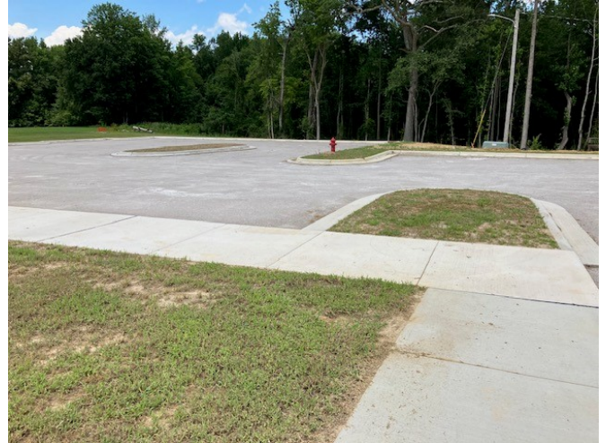
The parking lot is ready to be paved.
