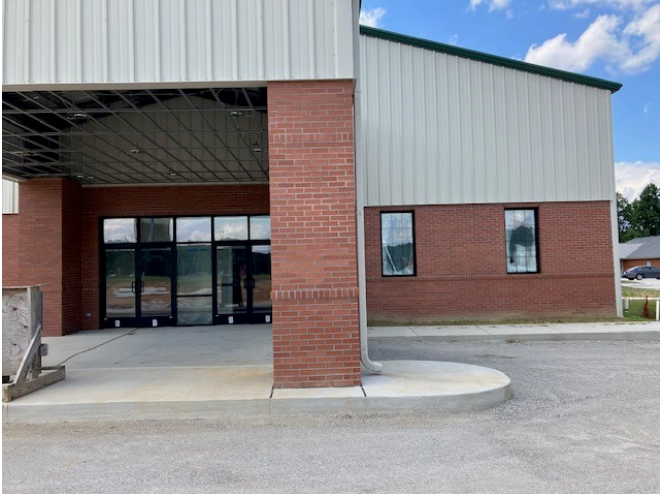
The front doors and windows are in!
